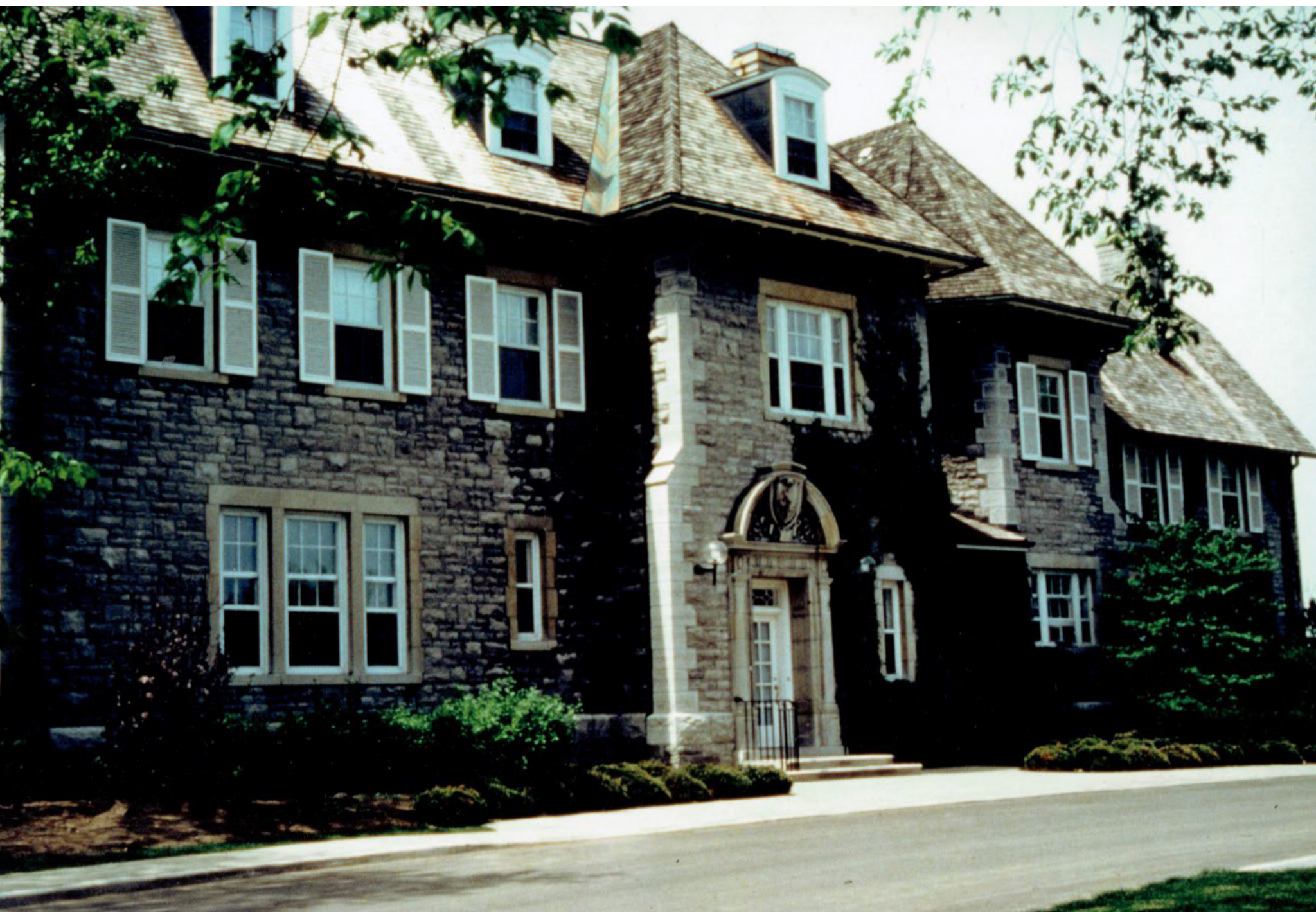
The traditional home of Canada's prime minister, 24 Sussex Dr., has sat empty since Justin Trudeau was first elected in 2015.
